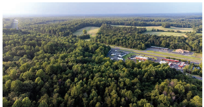
The proposed site of another data center. © Matthew Hartwig, American Battlefield Trust
