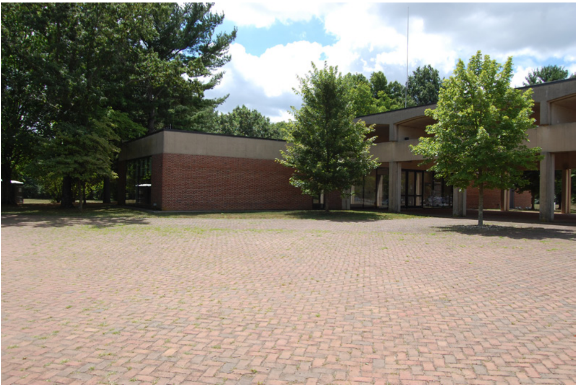
Figure 24: The previous building and bridge occupy one side of the brick plaza. JGWA 2022.
