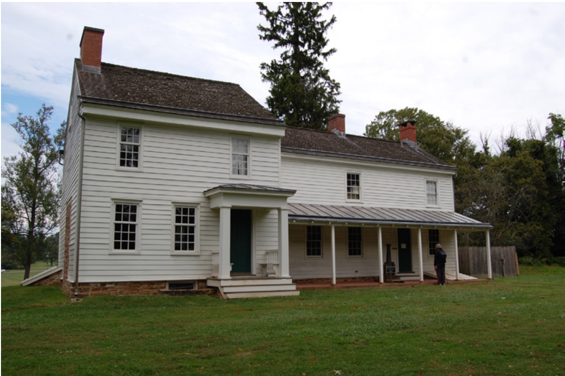
Figure 2: At the time of the Battle, the south facade of the house, the main entrance, faced the Sawmill Road, now gone. The Greek Revival stoop on the taller portion of the building and the two-story wing with piazza to the right are 19th century additions. JGWA 2022
