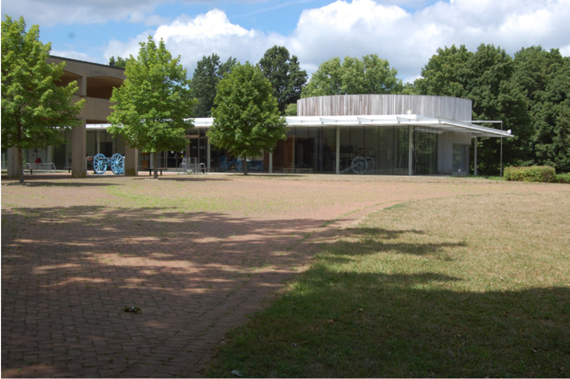
Figure 21: The tall space of the theater projects above the roof in a drum. The deep overhangs shade the windows to limit reflections when looking out, and to reduce heat gain. JGWA 2022.
