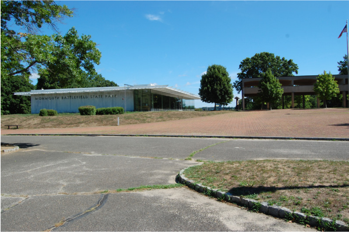
Figure 19: The new visitor center addition to the left faces the bridge and pavilion of the previous facility to the right. JGWA 2022.
