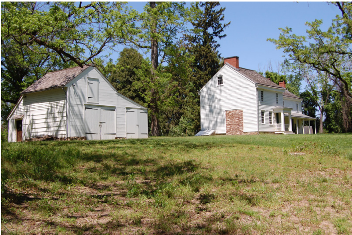
Figure 6: In a view from the southwest, the shed sits to the left of the Thomas Clarke House. JGWA 2023
